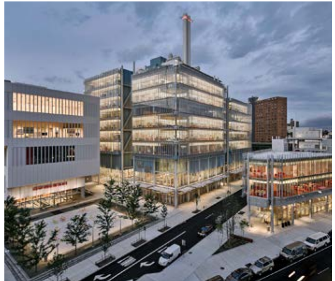
Mueser Rutledge Consulting Engineers Columbia University's Manhattanville Campus 2020 EEA Honor Award winning project
