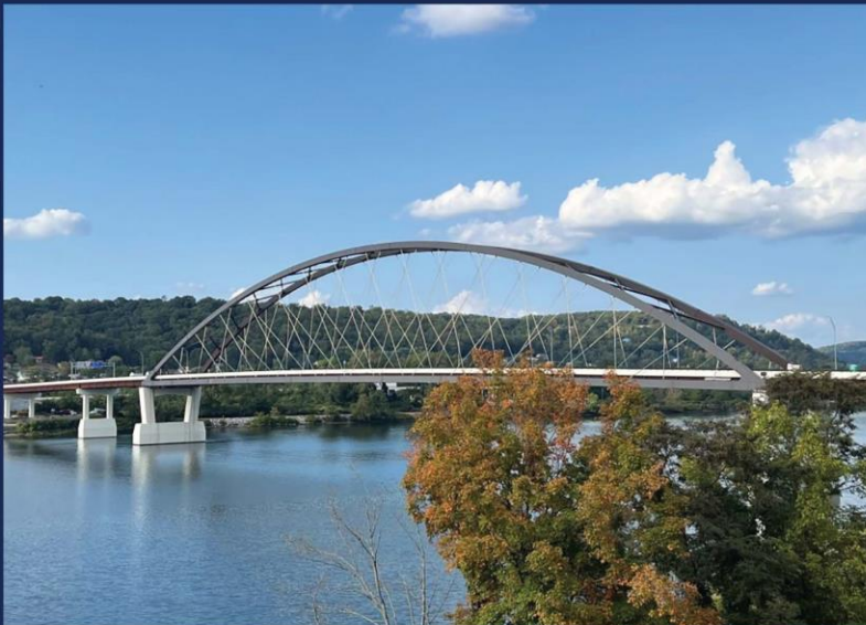
Completed Bridge Connecting Wellsburg, West Virginia and Brilliant, Ohio
