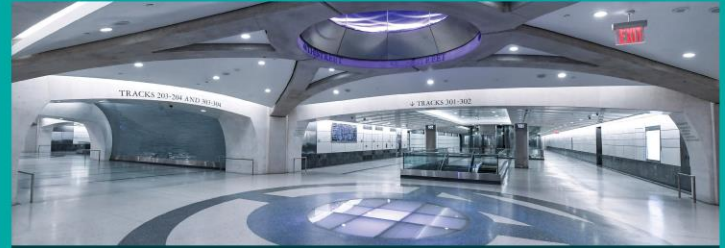
Completed station, mezzanine level. The station mezzanine levels allow for passenger flow between the two station caverns and up to the concourse level.
