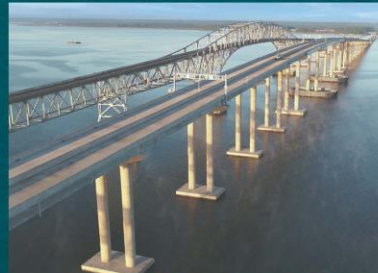
The innovative bridge design incorporated efficient and cost-effective span lengths that took into account: repetitive and fast construction techniques; simplified future maintenance inspection details; and minimized total cost of ownership for the 100-year service life.
