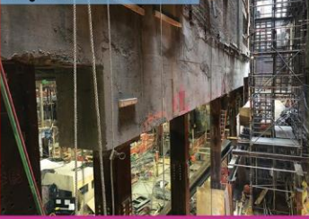
Ring Beam—After Theater Lift
