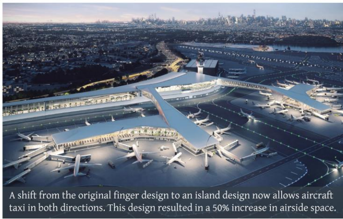
View of Pedestrian Bridge B which connects the New Terminal B Headhouse to the Island Concourse B from an airside vantage point. This element allows for planes to taxi in either direction from each gate.
