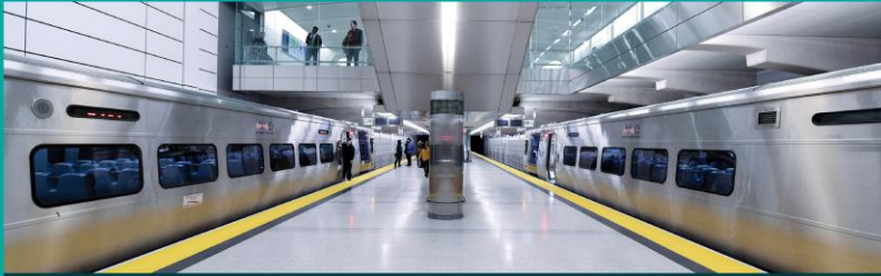
Completed station, lower platforms. The station and tail tracks allow for idling of up to 12 trains at a time. At 140-feet below Park Avenue, the caverns are the project's deepest excavations.
