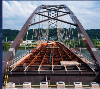
"Floating" Deck System in Arch Span
