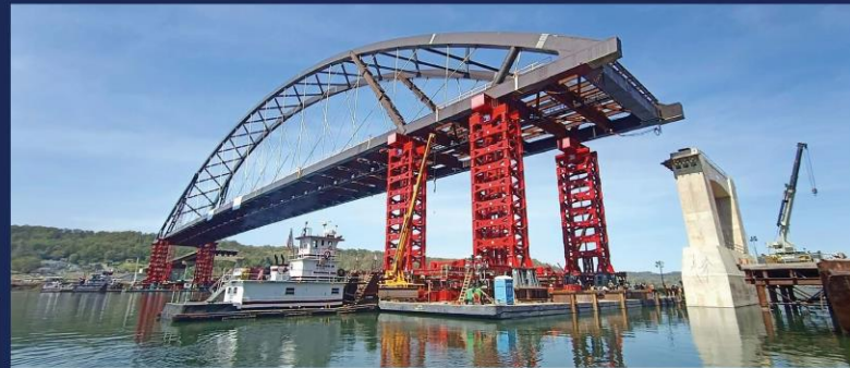
Innovative Approach: Steel Arch During Float-in Operation
