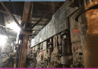
Ring Beam—Before Theater Lift
